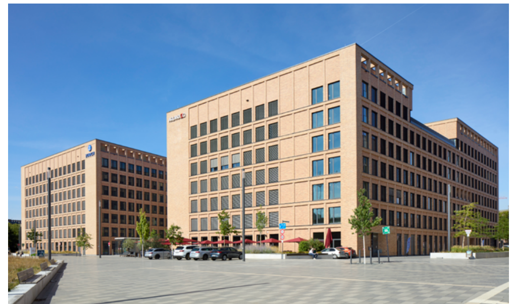
Further large units were taken up in the new MesseCity Köln buildings.
