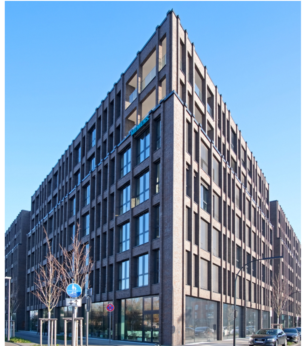
The large development area I/D Cologne constitutes a considerable expansion of the submarket of Mülheim. The existing focus on the creative and IT industries is increasingly complemented by big corporations and public authorities.
