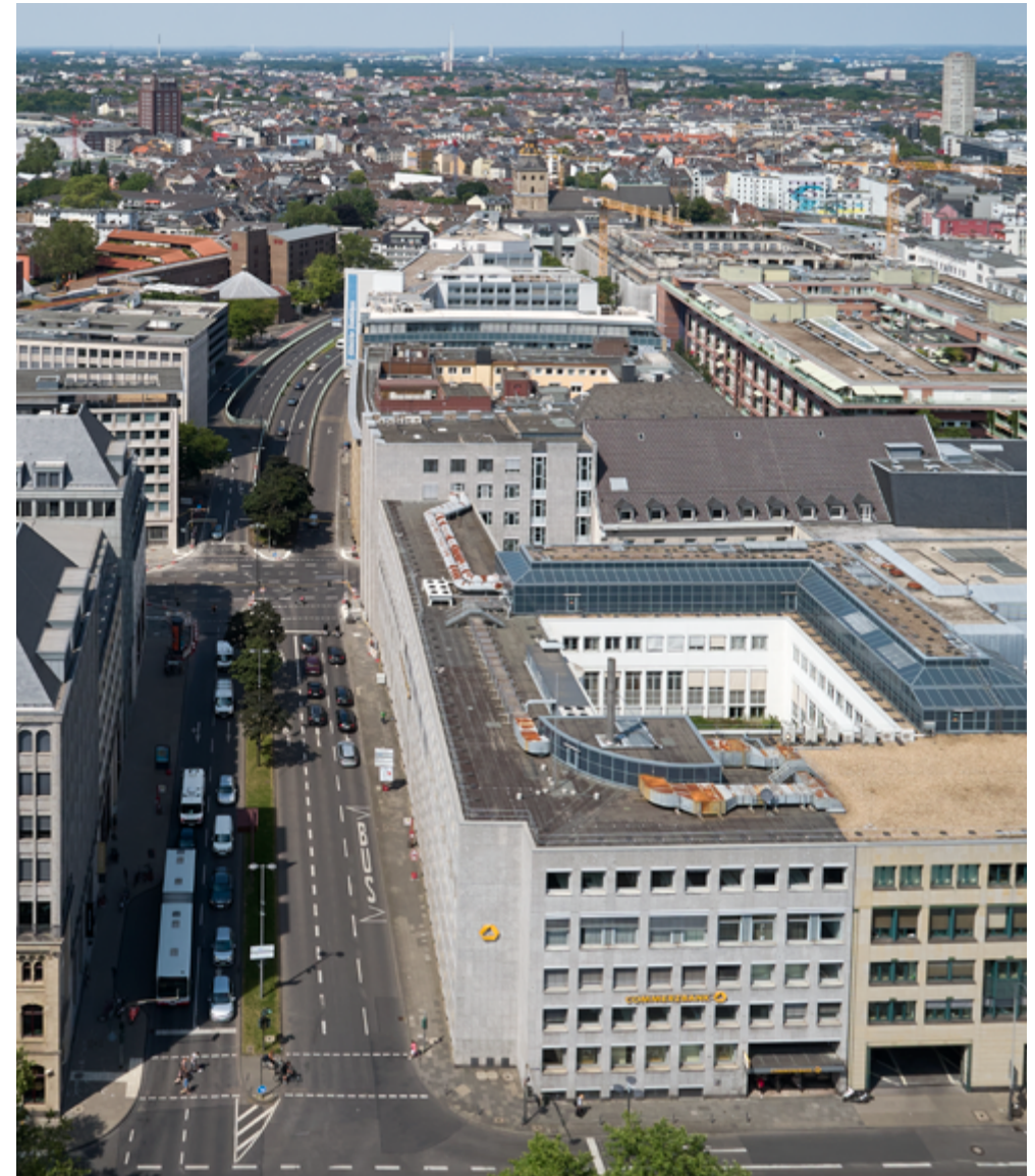
To be able to refurbish its headquarters in the banking quarter, the Cologne Chamber of Industry and Commerce picked up a unit in the nearby office building Unter Sachsenhausen 5-7 that was previously used by Commerzbank.
